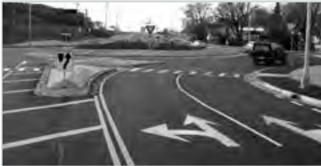
Figure 2.11a: WIS 30 and Thompson Drive in Madison
