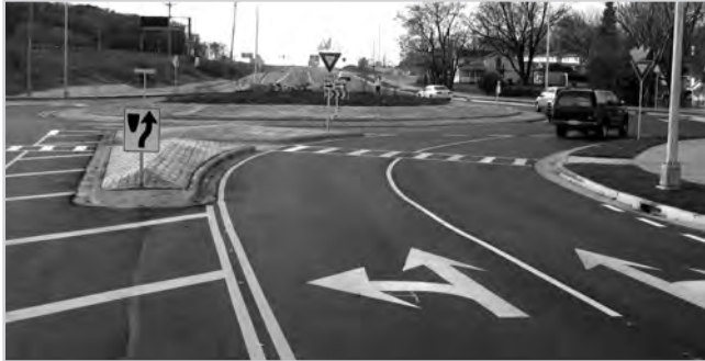
Figure 2.11a: WIS 30 and Thompson Drive in Madison
