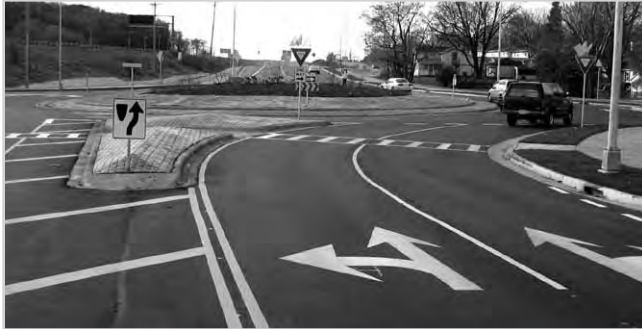
Figure 2.11a: WIS 30 and Thompson Drive in Madison
