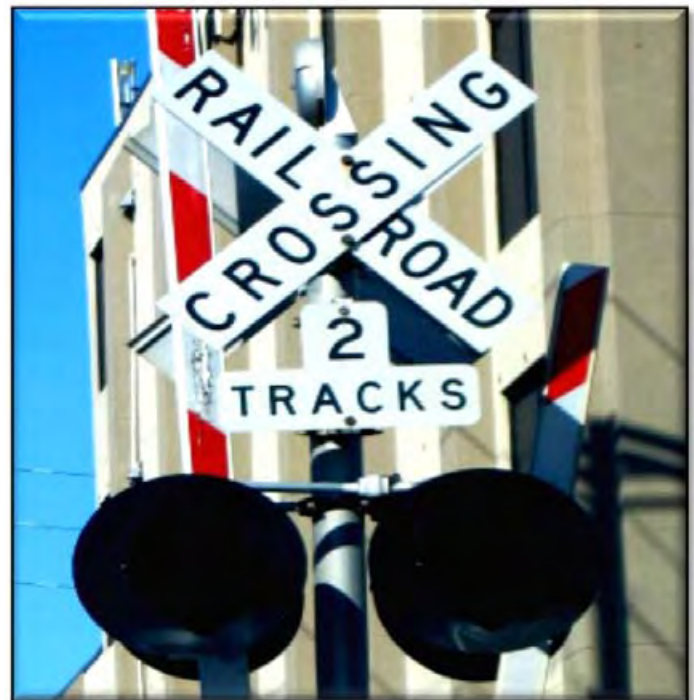
Figure 2.17 Railroad Crossing Gate and Light With Multiple Track Warning Sign
